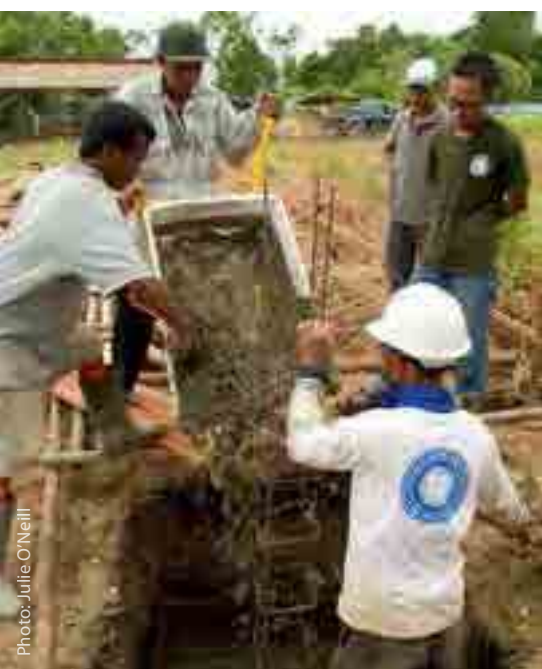
Laying the foundations for the new centre
